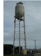
Elevated Water Tank
